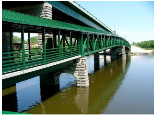
Photo 1, Above: Customrock Formliner “Random Cut Stone” pattern used on beam and truss style pedestrian bridge in Fox River, IL.
