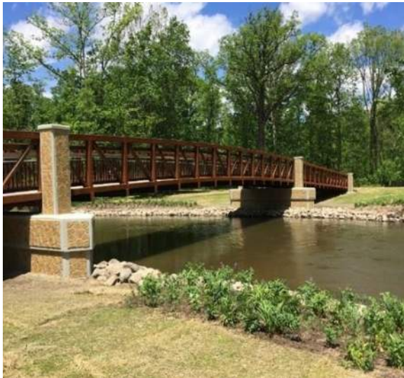
Photo 2, Above: Truss style bridge stone pattern and stained concrete coloration/pattern at Dodge Park, Sterling Heights, MI.
