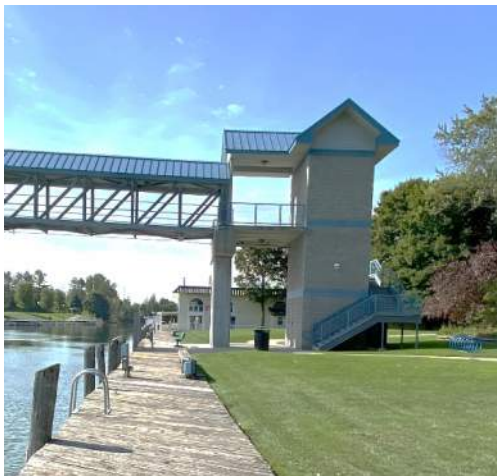
Second Floor landing is supported by CMU wall of elev/stair tower.
